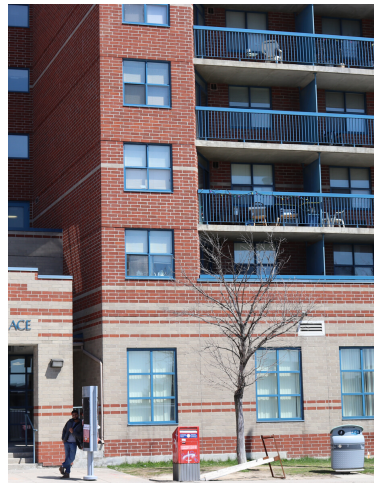
WALTON PLACE 12 accessible apartments integrated into the Walton Place
